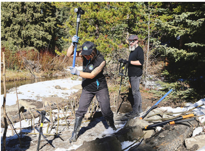
Staking willows to restore streambanks and reduce erosion at Pasque Creek.
