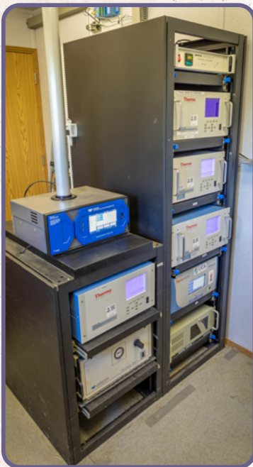
Instrument rack at Cold Lake
