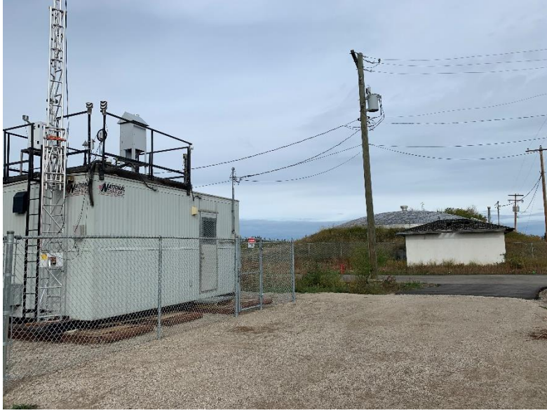
Exterior (AQM Shelter)
